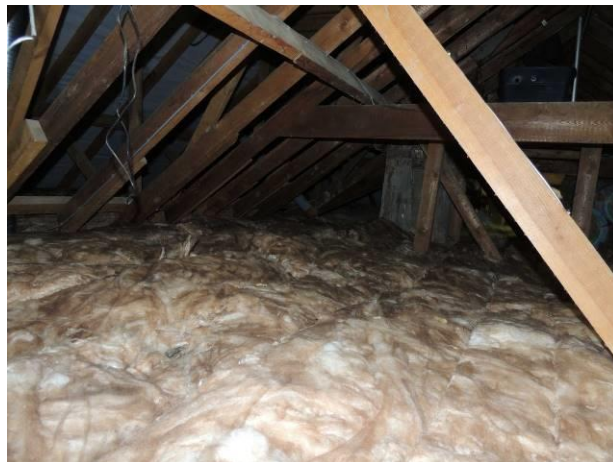
Note lack of evidence of bats on loft insulation
