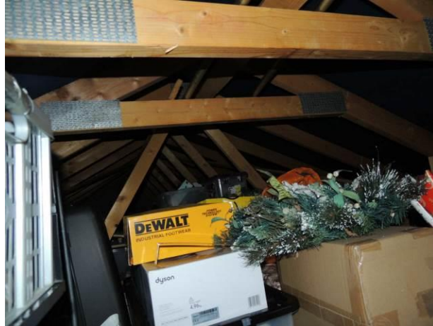
Note shallow-pitched roof void
