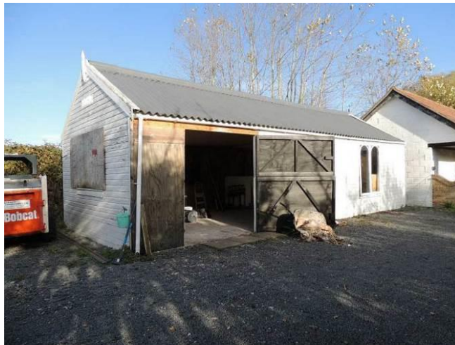
South-eastern elevation of 'The Chapel'
