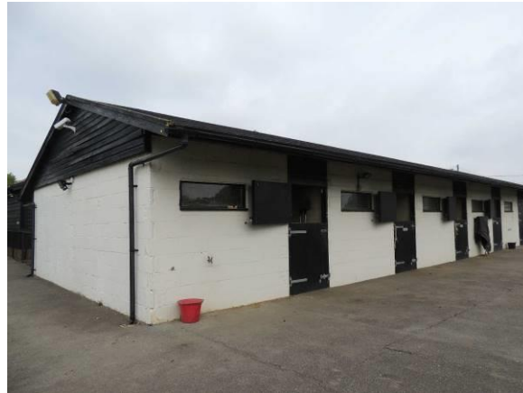
North-western and north-eastern (gabled) elevations
