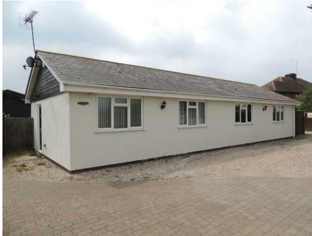
Northern elevation. Note tight seal to roof slates
