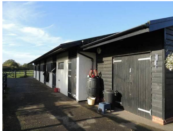
South-eastern elevation of the stables
