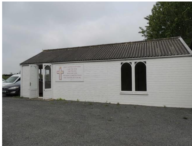
South-eastern elevation of 'The Chapel'
