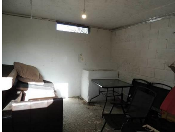
Interior of stable bay
