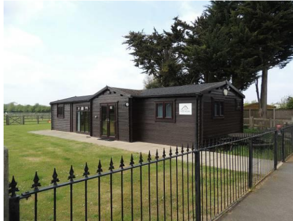
North-eastern (gabled) and south-eastern elevations
