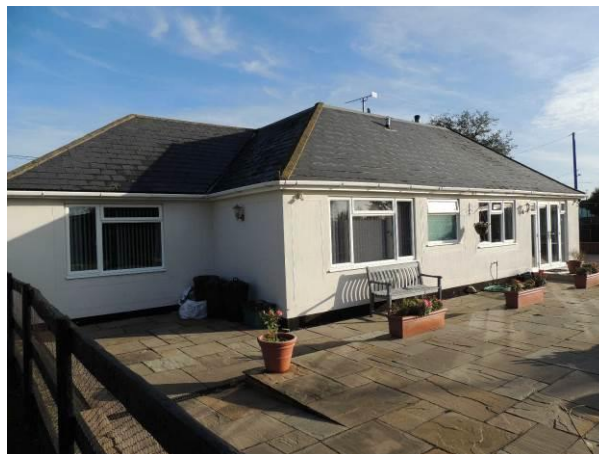
Southern elevation. Note tight seal to roof slates
