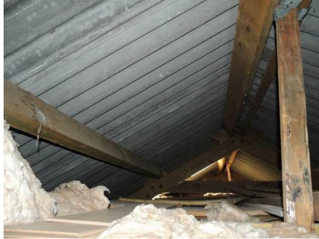
Note lack of evidence of bats in shallow-pitched loft
