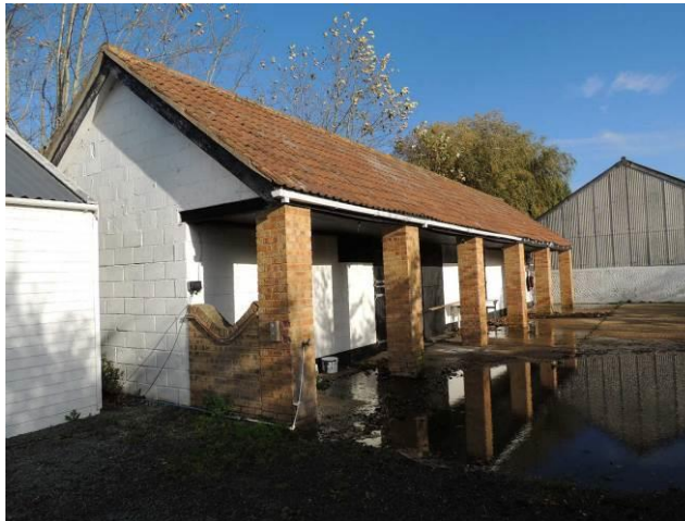
South-eastern and south-western (gabled) elevations
