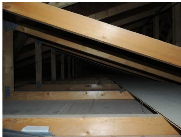
Note lack of evidence of bats in roof void of stables
