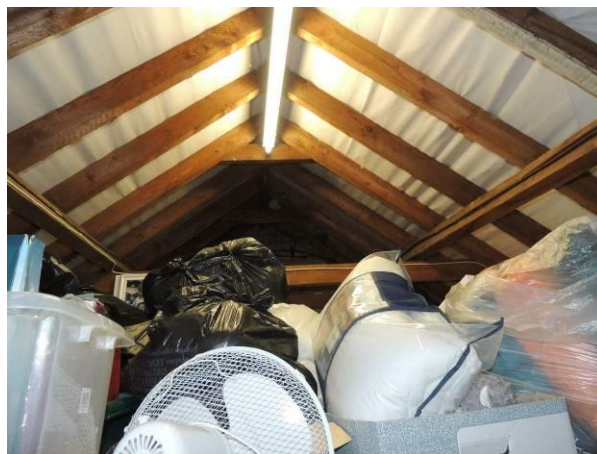
Note shallow-pitched roof void
