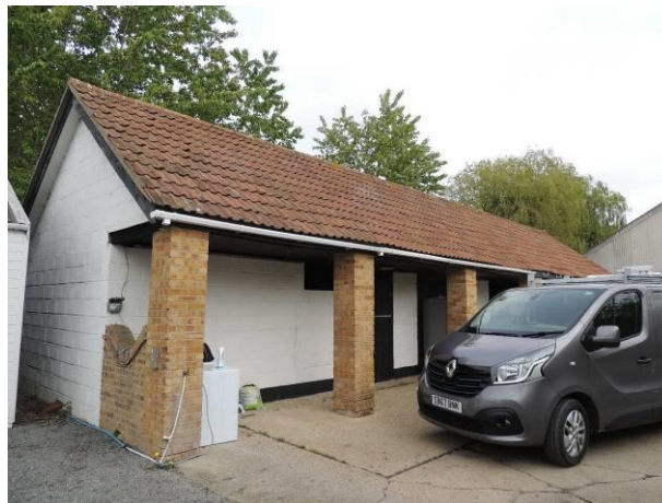
South-eastern and south-western (gabled) elevations
